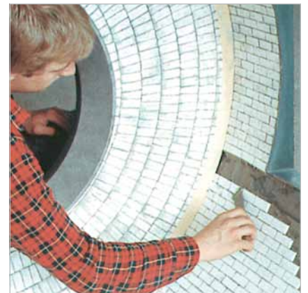
KALOCER mosaics of 1.5 to 12 mm allow flexible use; they are fixed by KALFIX epoxy setting compound
