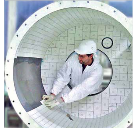
Lining a cyclone inlet with KALOCER; the arch shape enables fixing radial shaped elements in KALFIX setting compound whereas the headwall requires mechanical fixing by means of weld sleeves and ceramic caps
