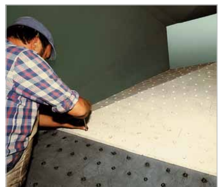
Mechanical fixing to meet special requirements
