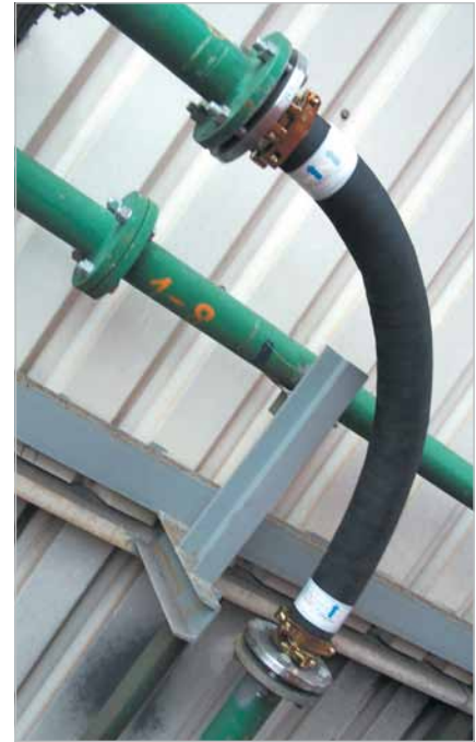
KALFLEX used as flexible pipe bend
