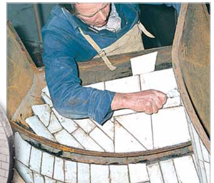
Chutes lined with KALCERAM are a solution that lasts, e.g. for bag loading systems in cement plants
