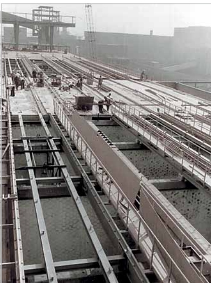
Raw material hopper in a German blast furnace plant
