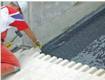
High temperature KALCERAM-K chute in a coking plant provides good sliding properties even at high temperatures
