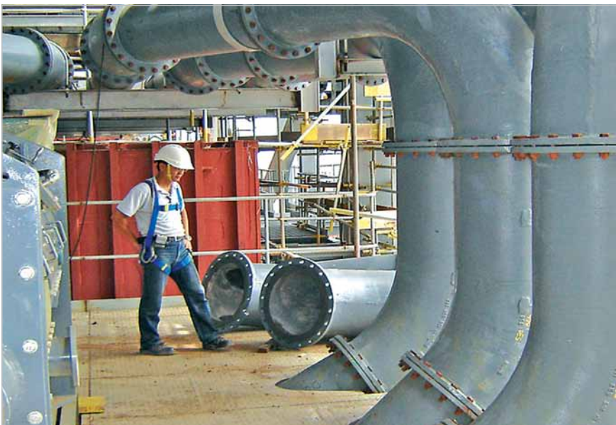
Typical applications of KALMETALL-C hard casting are pipe systems; here a pulverized coal pipe of a power station in South East Asia
