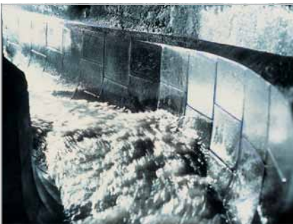
Flumes and hoppers of any shape can be lined with abrasion resistant ABRESIST
