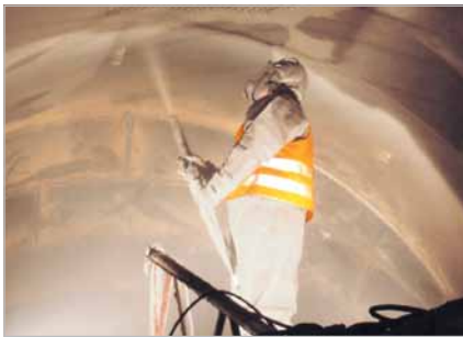
Overhead working possible without difficulty
