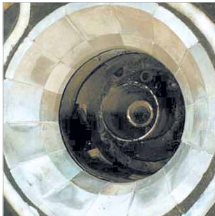
Burner cone for a power station made of KALSICA-N
