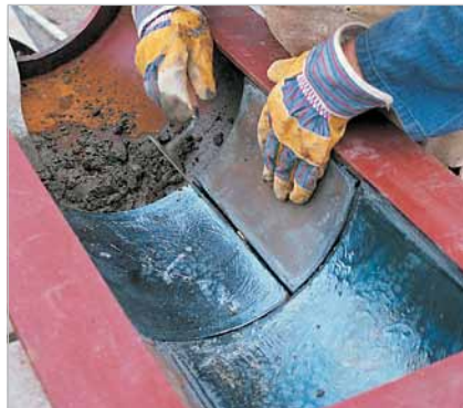
Setting in cement mortar
